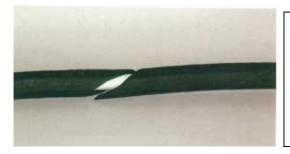
For conduit splice: the conduit ends must be cut at an angle between 30 and 45 degrees from the center line of the conduit and butted together tightly. Secure in place with RM Tape and proceed to jacketing Repair.
