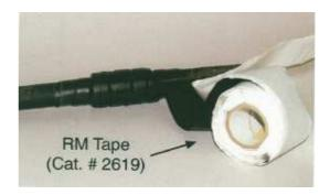
**For conduit repair**: Minimum wall thickness of conduit and sleeve must be 1/4 inch. If a section of damage conduit is missing, this wall thickness may be achieved by placing a patch of RM Tape under the sleeve, secure it in place with RM Tape (Cat # 2619) and proceed to jacketing repair.
